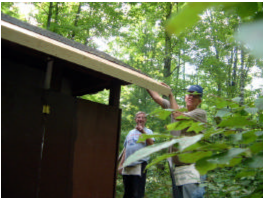
Harvey Bruecks and George Wagner install new fascia on Latrine dutv.
