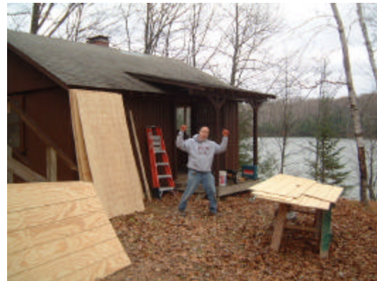
Scott Smith cutting up at Cabin 2
