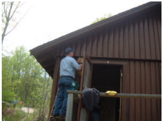
Larry Neuman installs a new outside light at Cabin 4
