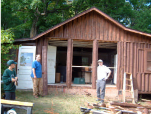
Greg and Fred at work on rehabbing cabin 7
