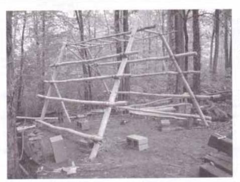
This is the frame for the new Wigwam to be used near the bowl. This will replace the tipi that stood for years on the north end of the bowl. There will be a sheathing of bark that will enclose the frame. The bark is made of a synthetic material but looks exactly like bark.
